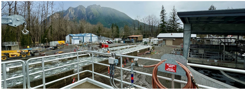
Figure 1 Wastewater Treatment Plant (2024)
