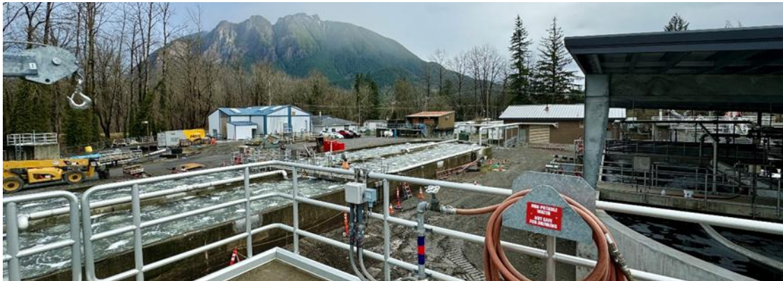
Figure 1 Wastewater Treatment Plant (2024)
