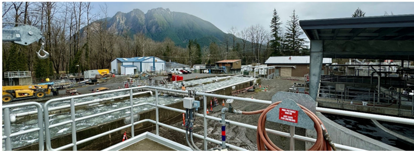
Figure 1 Wastewater Treatment Plant (2024)
